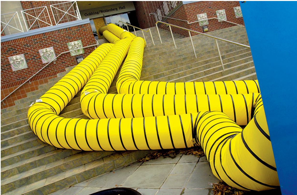
An industrial dehumidifier pumps cool, dry air into Goldring/Woldenberg Hall to prevent the spread of mold, Sept. 29, 2005. Photo by Paula Burch-Celentano.
